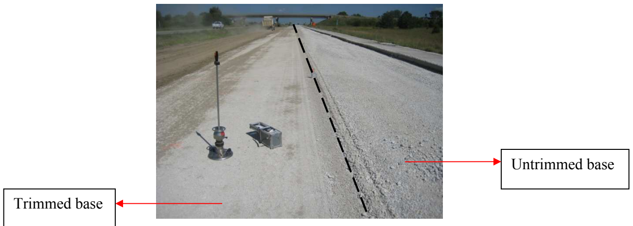
Figure 24. Trimmed base (left) and untrimmed base (right) for I-35 Iowa
