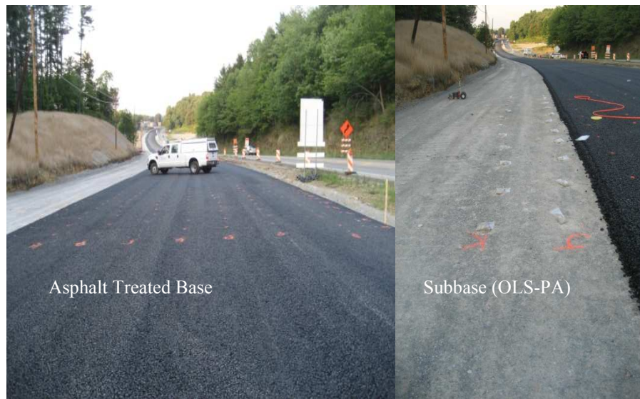
Figure 41. Overview for test bed (left) and subbase test location asphalt treated base on US-22, Pennsylvania
