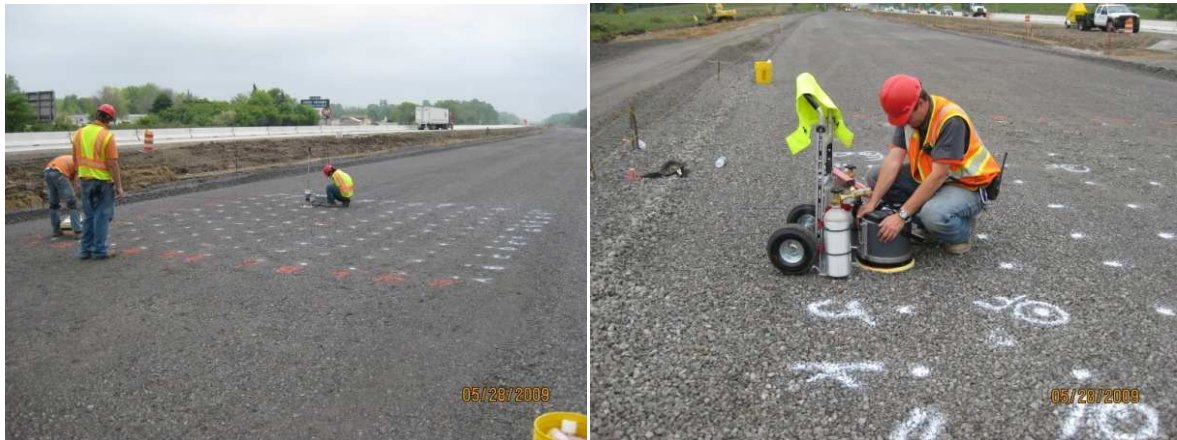
Figure 31. Overview for test bed (left) and GPT in situ testing on I-94, Michigan
