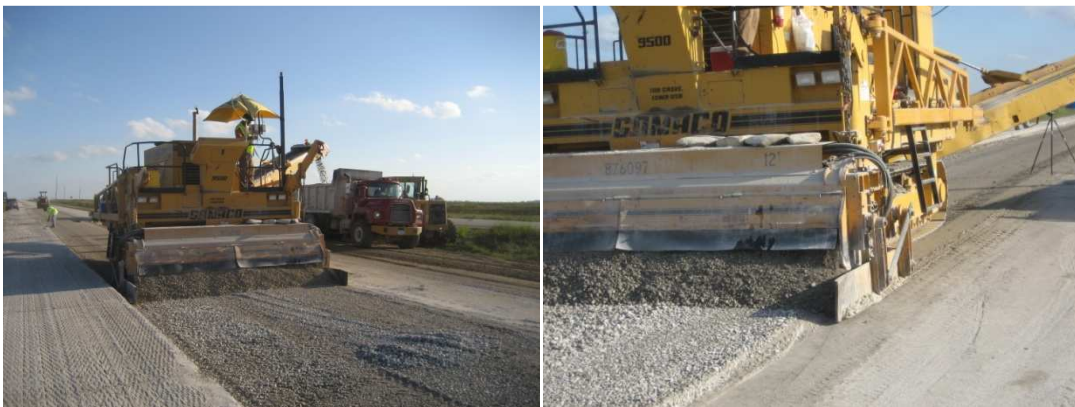
Figure 25. Trimming process for I-35 Iowa
